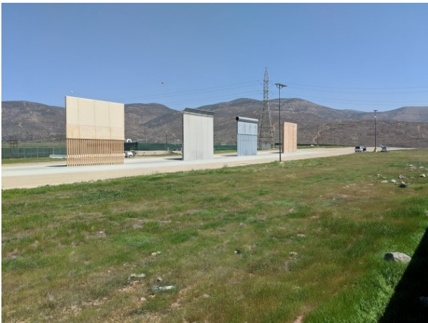
Two photos of the wall prototypes.
